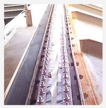
DE**KOM**TE recommends the retrofit of additional water barriers, drains and integrated flow plate systems. These give the security of a cleaner, longer functioning expansion joint by eliminating the build-up of water, deposits and debris from inside the joint space.
