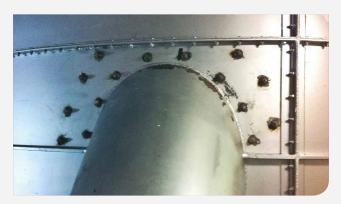
During an annual inspection, one of our customers discovered they had poor insulation in the internal liner plates of their GT Exhaust duct. The plant had repaired the liner plate issues and renewed the insulation, but the location was still showing hotspots.
